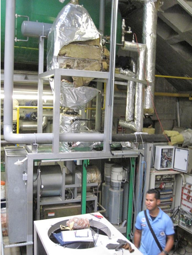
Installation of the microtrigeneration system in Districlima (Barcelona)
