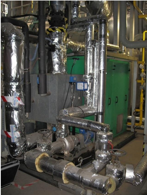
Installation of the microtrigeneration system in Districlima (Barcelona)
