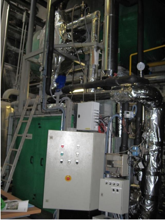
Installation of the microtrigeneration system in Districlima (Barcelona)
